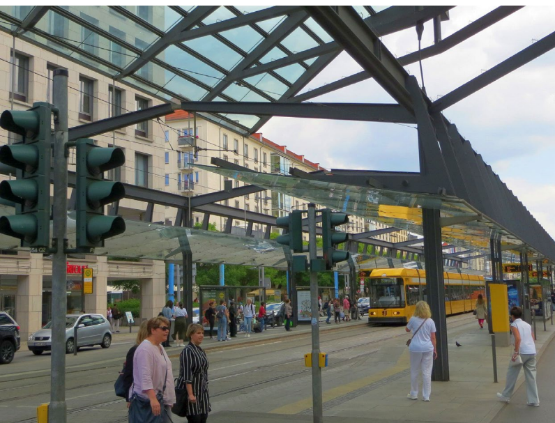
Photo credit: Douglas J. Cross, covered passenger waiting areas in Dresden, Germany.
