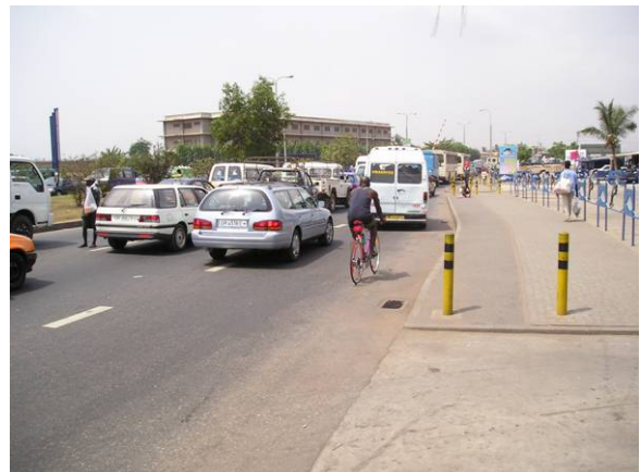
Figure 6: Drop-kerb across path Surface-dressed strip along the kerb meant as cycle track. Brick pavement to the right meant as walkway.
