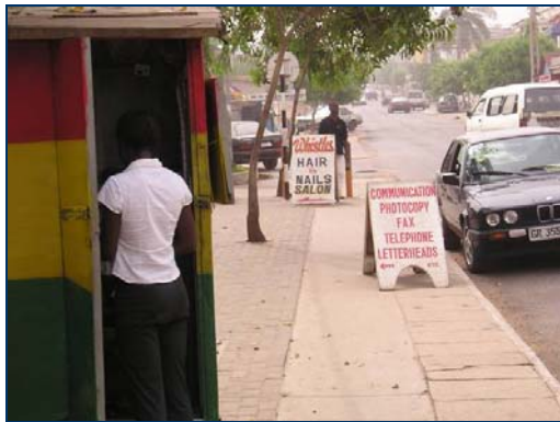
Figure 3: Unused Nime - CBD cycle path section (2004). Slab cover of blocked drain. This, together with the adjacent strip of bitumen surface dressing, constitute the cycle track. Brick pavement to the left meant as walkway
