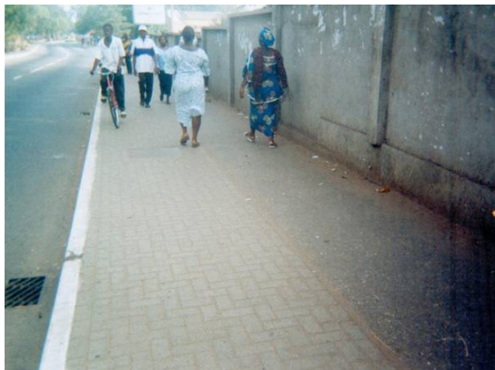
Figure 7: Walkway between carriageway and cycle track
