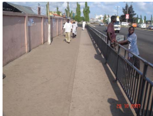
Figure 8: Combined walkway/cycle track, separated from carriageway by a fence. Between Circle and Obetsebi Circle, path 3 (2007)
