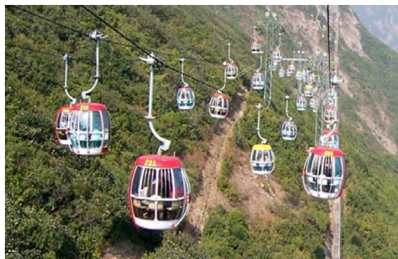
Plate 18: Hong Kong Ocean Park Gondolas - showing two adjacent lines attached to the same station
