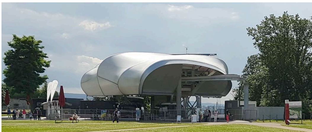
Plate 13: Koblenz ART stations blended with the surroundings Source: Author
