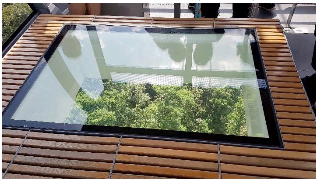
Glass floor window, Koblenz ART cabin 17. Source: Author
