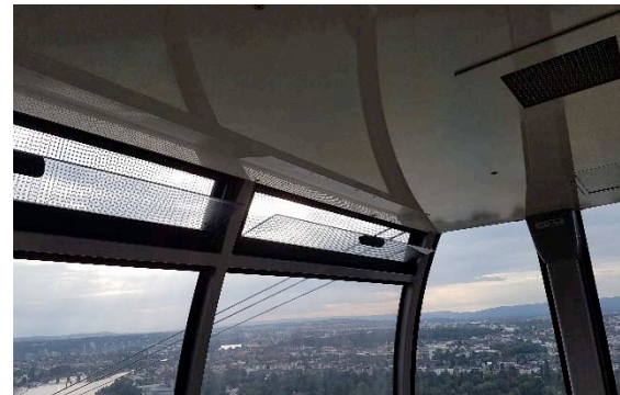
Koblenz ART cabins - ventilation windows Source: Author
